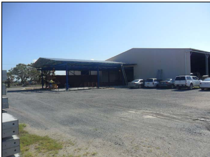
Plate 2 – View looking towards the manufacturing shed from the north east
